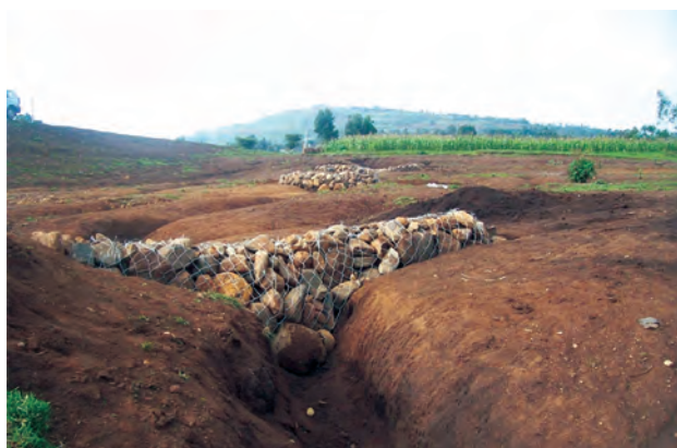
Figure 4 Gully Plugging.
